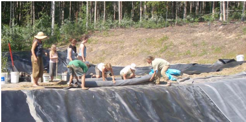
Crew relining new pond
